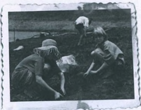
All helped to grass the spillway of the new dam.
