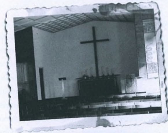
The school chapel interior. The chapel was built in 1960
