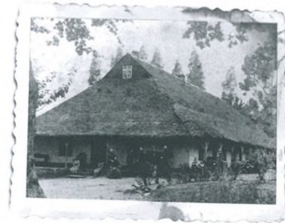
One of the very first photographs taken of the Mission House, which now has a corrugated iron roof.
